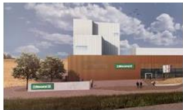
Haag, Austria (under construction, 2020)
